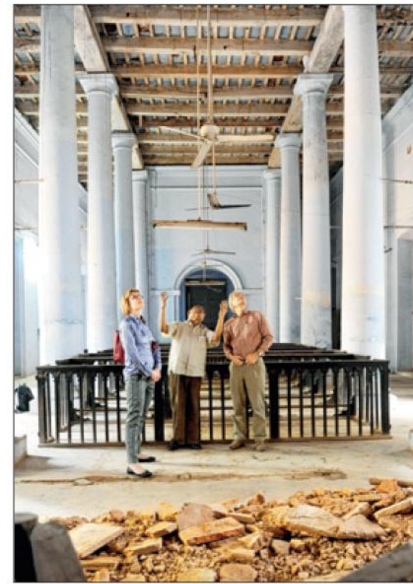
Bente Wolff, conservation architect Manish Chakraborti and Flemming Aalund survey the heavily damaged St. Olav's Church
